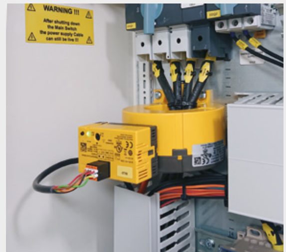
CTUB100 series measuring current transformer in the distribution units
